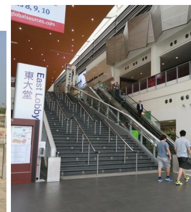
Escalators 扶手電梯
