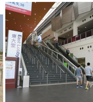
Escalators 扶手電梯
